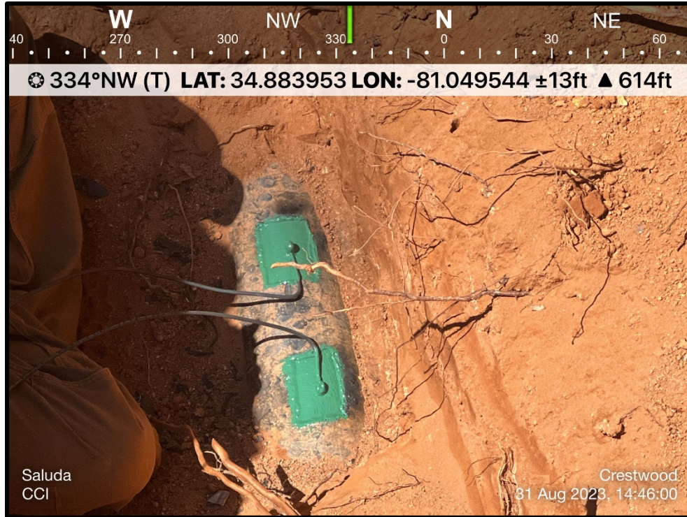
S-2: Epoxy mastic coating applied to weld area.
