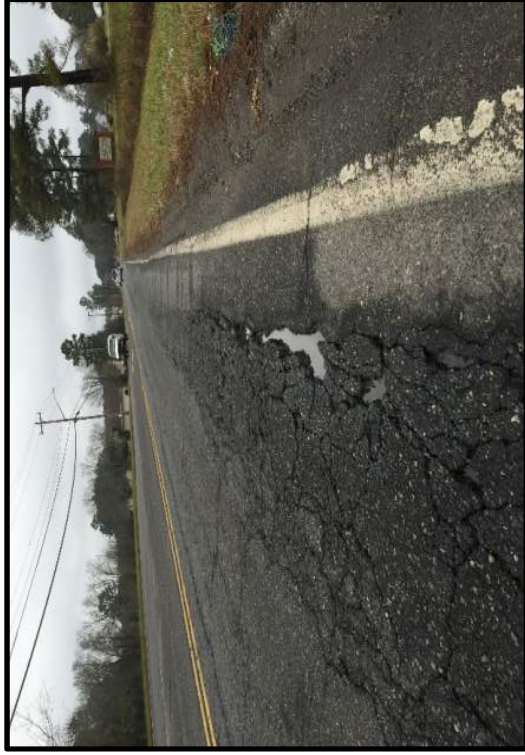
Looking southwest from about station 110+00 SC72. Note Distressed pavement
