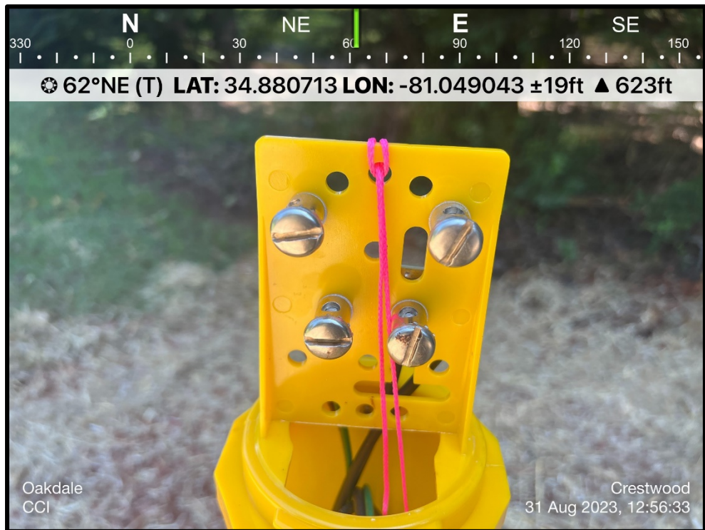
O-4: Magnet on a lanyard suspended inside the test station.
